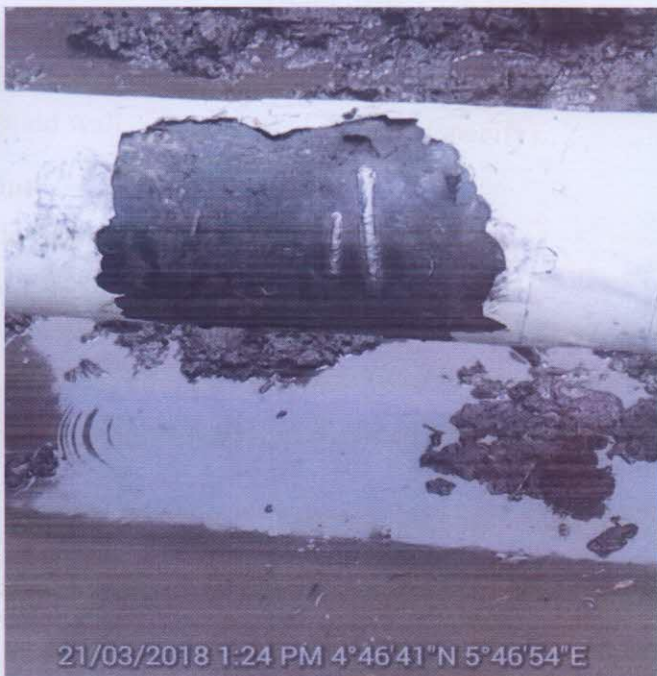
Fig D: Incident facility during repair
