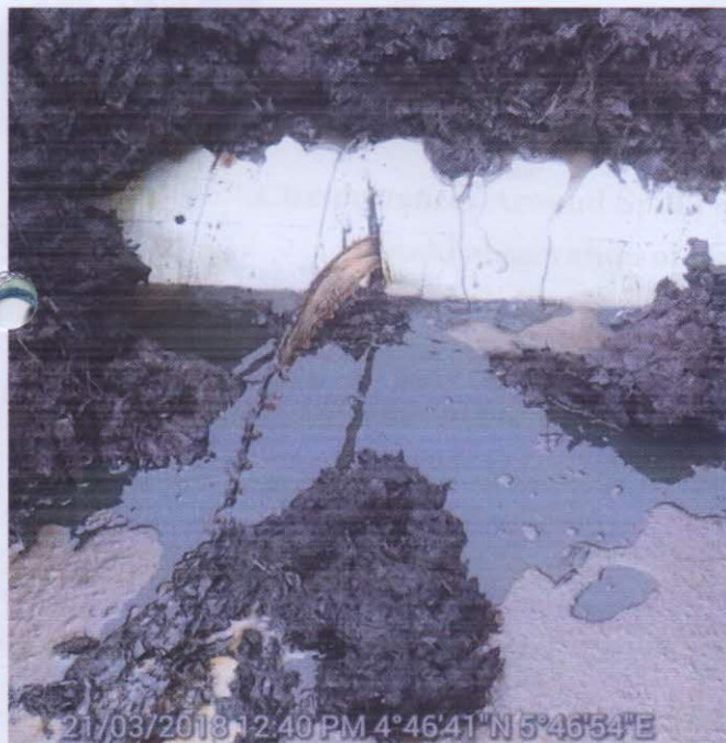
Fig C: Incident Facility after excavation
